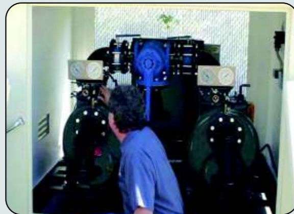
Duplex lift stations packaged complete with controls and piping in easy access fiberglass enclosures
